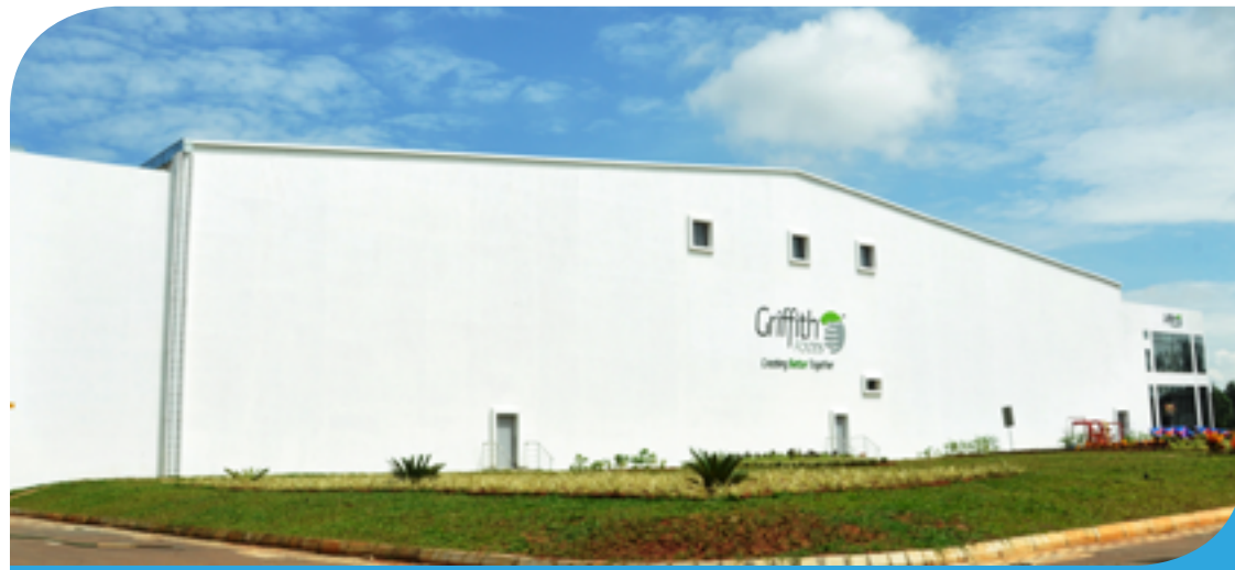
Griffith India's new manufacturing plant is now fully operational
