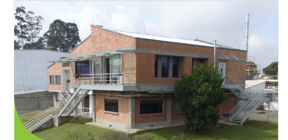
Griffith Foods Colombia's new Research and Development center is LEED Gold Certified by the US Green Building Council (USGBC)
